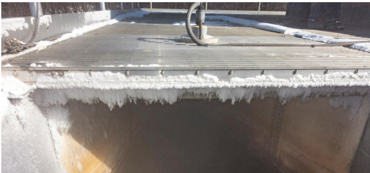
The influent channel gets frosty during the cold winter months, making it a challenge for some level measurement instrumentation to make a reliable, accurate measurement in the flume.
