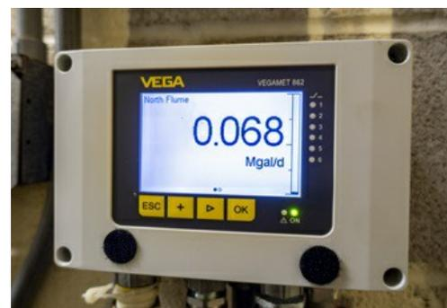
The VEGAMET 862 controller displays the radar sensor's measurement in millions of gallons per day using a brightly lit, easy-to-read LED screen.
