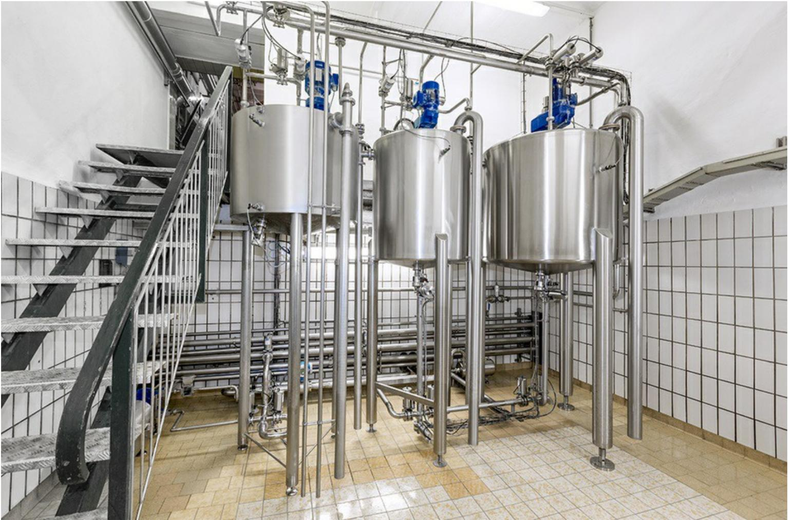
In the beer filtration process, VEGABAR ensures exact quantities in the kieselguhr dosing containers.
