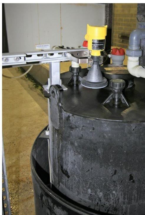
Radar sensors are mounted above all small day tanks containing acids and alkalis. They measure the liquid level from the outside
