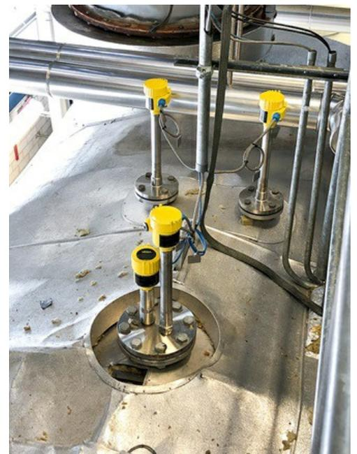
The redundant measurement ensures that the water level stays in the optimum range.
