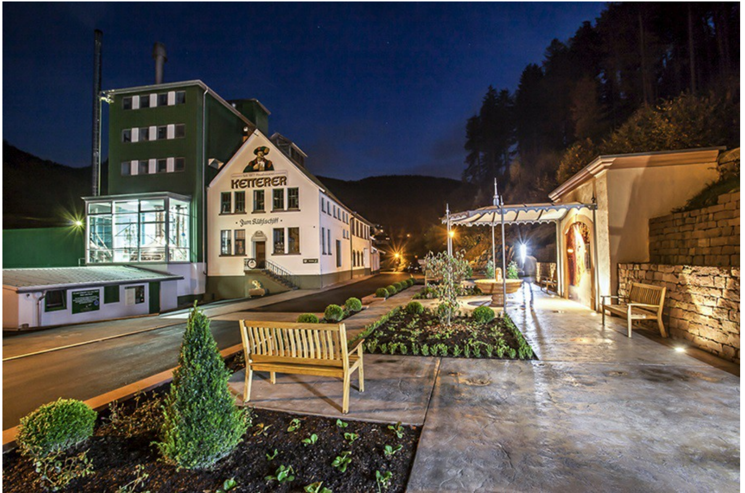
Front façade of the Ketterer brewery in Hornberg.
