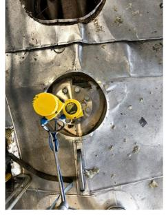
Mounted on a shared flange, both the transmitter and point level switch instruments confirm each other's results.
