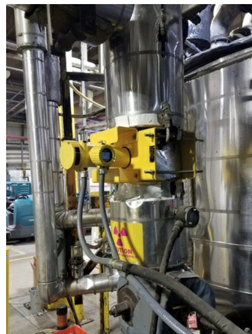
A MiniTrac 31 measures the density of contents traveling vertically in a pipe.
