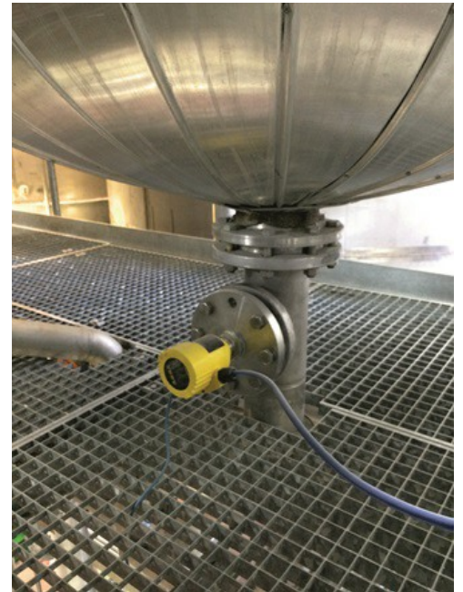
Electronic differential pressure measurement of a primary sensor in a distillation tank.
