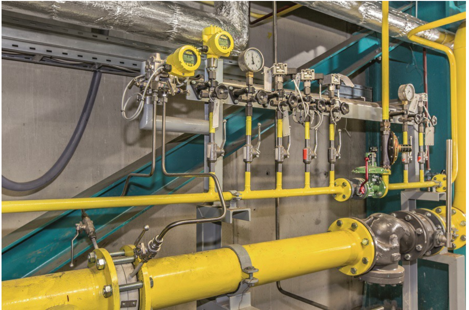
Flow measurement via an orifice plate and mechanical differential pressure. The static pressure is measured by an additional sensor.
