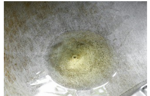
Oil on the tank floor. At low levels, it is very difficult to measure oils or other liquids accurately.
