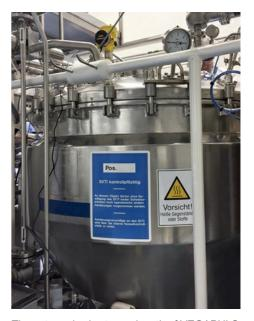
The extremely short wavelength of VEGAPULS 64 radar sensors enables a high-precision level control throughout the entire production process.
