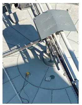
When measuring inside the tall, slender silos, anything that gets in the way, like internal fixtures and struts, are a big challenge. The precise focussing of VEGAPULS 69 sensors helps separate the measuring signal from interference signals.
