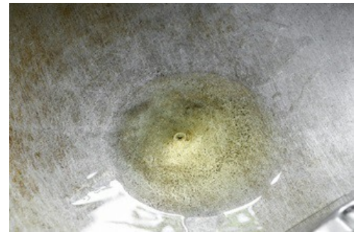
Oil on the tank floor. At low levels, it is very difficult to measure oils or other liquids accurately.
