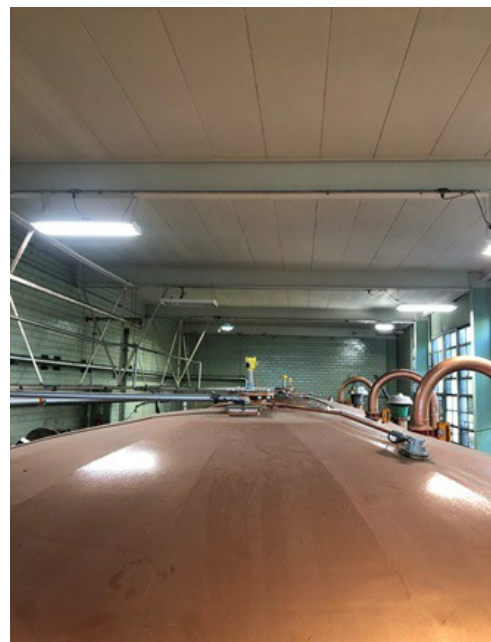
VEGAPULS 64 radar sensors with 80 GHz technology measure level in multiple fermenter vessels in the fermentation room.
