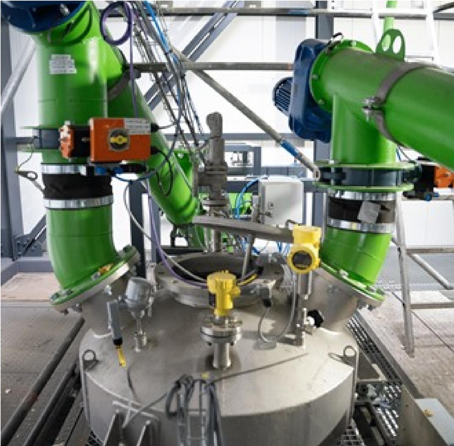
VEGA sensors monitor the pressures and filling levels throughout the entire process.
