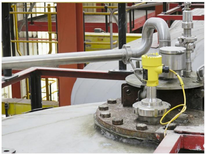
VEGAPULS 64 has a hygienically flawless antenna connection and can be mounted front flush.
