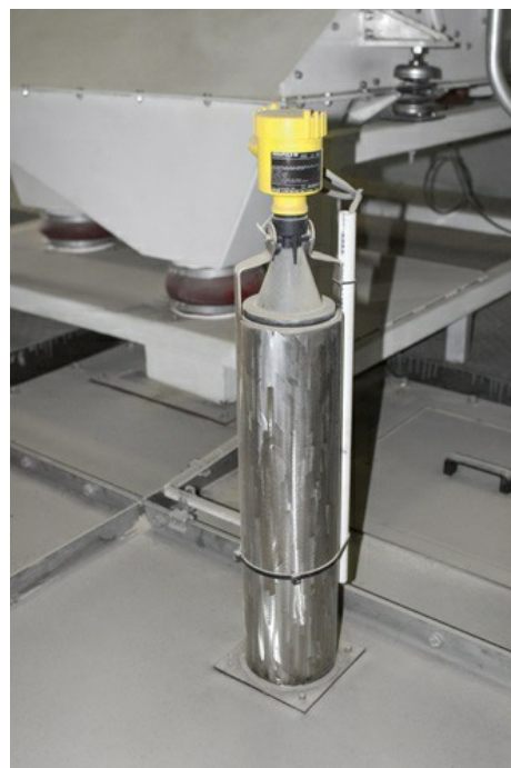
Despite the significantly shorter wavelength of VEGAPULS 69, the sensor is very insensitive to deposits.
