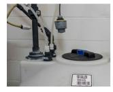
Operators had never been able to maximize the use of the fluoride day tank because of the way ultrasonic technology works. The installed transmitter had a near zone, or "dead band," spanning 12 inches directly below it, so the tank could never be filled to the top. Plus, condensation on the sensor routinely caused measurement errors. Replacing the ultrasonic transmitter with an 80 GHz radar sensor – the VEGAPULS C 21 – eliminated these problems, and installation was easy.
