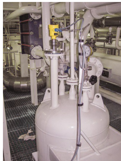
VEGAPULS 64 measures the level in a cooling system on board a gas tanker.
