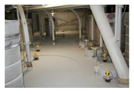
Every silo now has a VEGAPULS 69 that replaced the existing silo weighing system.
