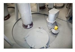
This photo shows how narrow the silos are and why VEGAPULS 69 performs so well. There is hardly any room for the sensor, yet its narrow beam angle allows it to work reliably in spite of that
