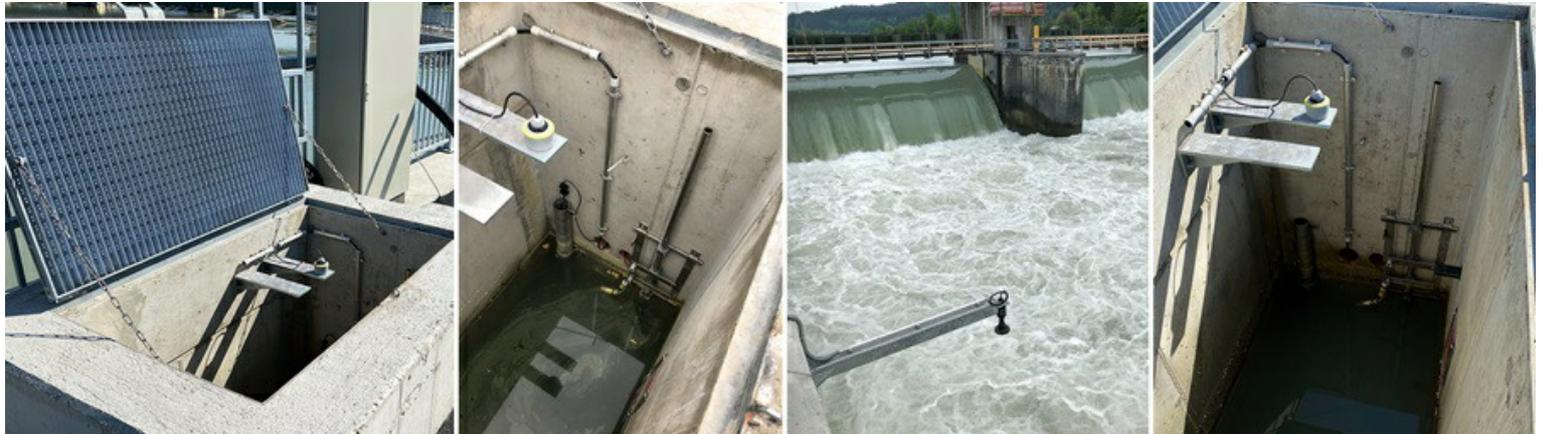
Although there is still some construction work to be done in Kirchbichl, the sensors have already passed their field test. Pairs of sensors from the new **VEGAPULS C 21** series are now continuously monitoring levels along the waterway: at the inlet channel, at the intermediate measuring point, at the forebay and in the downstream area below the turbine as well as in the pump shafts.
